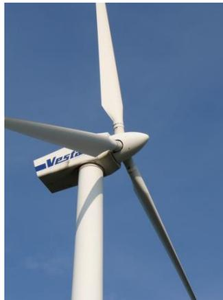
**Gambar 21.** Turbin Angin Sumbu Horizontal
