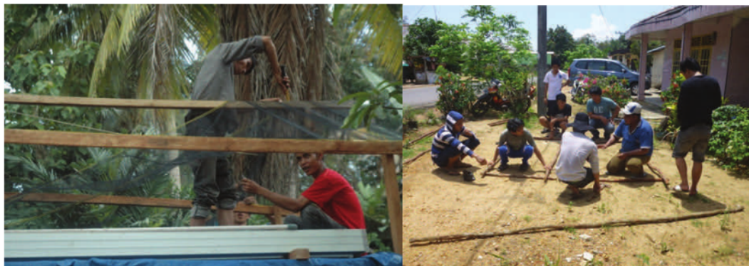
Figure 2. Preparation of Tarp Pond
