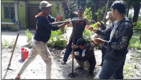
Gambar 11 Proses hand boring
