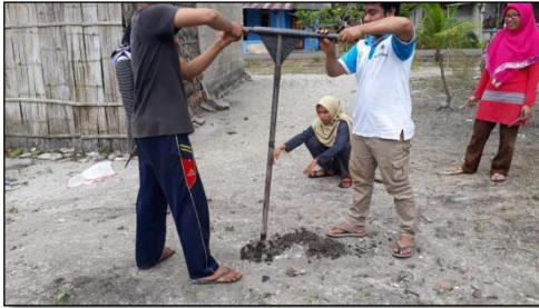
Gambar 38 Proses hand boring
