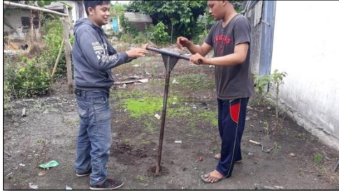
Gambar 31 Proses hand boring
