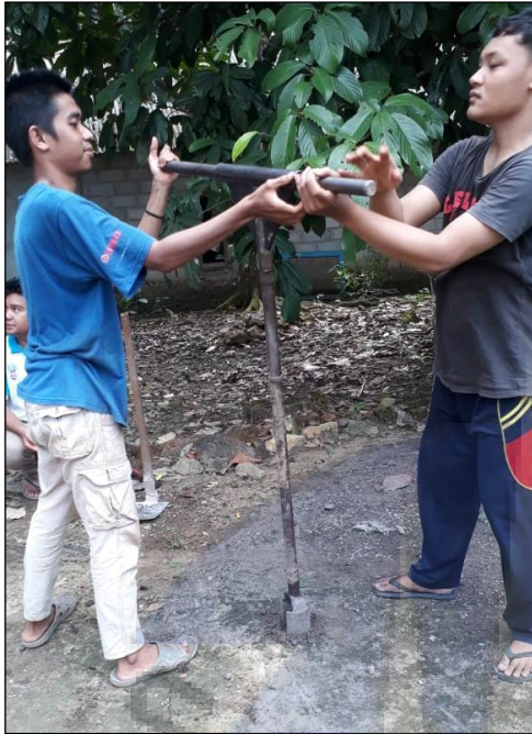
Gambar 24 Proses hand boring
