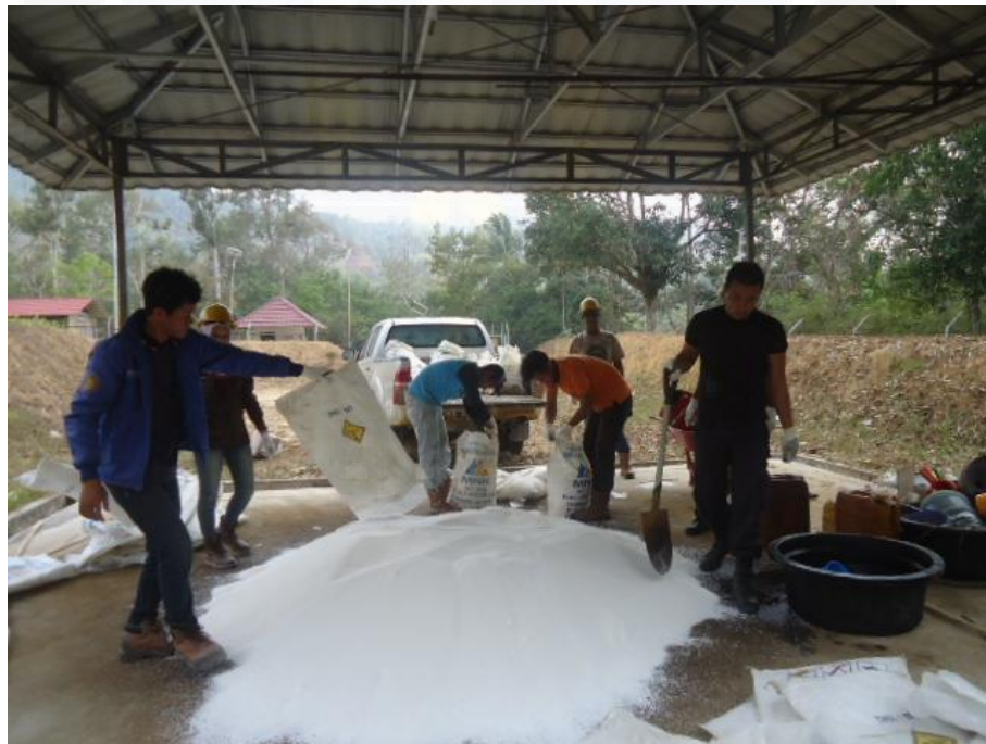
Gambar R.8 Kegiatan mixing Ammonium Nitrat dengan Fuel Oil
