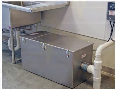
Gambar 5. 25 Grease Trap (Sumber: Pinterest, 2025)
