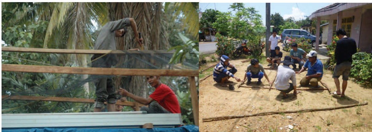
Figure 2. Preparation of Tarp Pond
