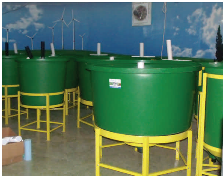
Assembly of the fish and filter tanks that will provide fresh fish and vegetables to the residents of the Survival Condo.
