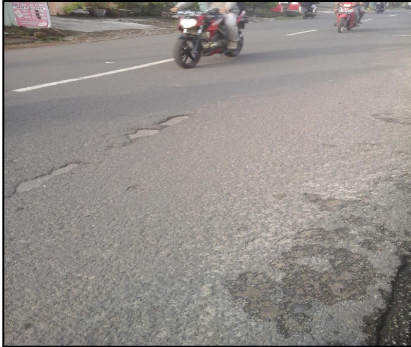
Gambar Kerusakan Keriting STA 0+092
